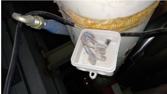
14.3.2018 open connection with dirt
