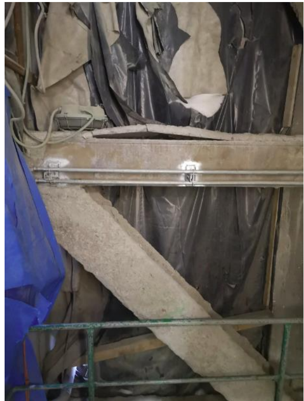
10.1.2019 bent Beam next to Turbine hall
