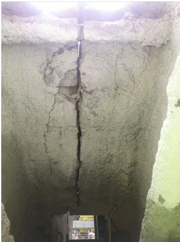
6.12.2018 Stairwell next to Turbine hall
