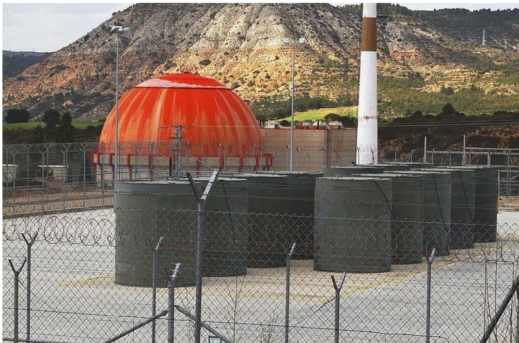
Figure 4.2-6. Outdoors spent fuel dry storage facility, José Cabrera nuclear power plant, Spain.
